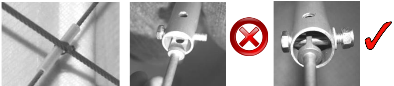
Figure 91 securing crossing cables, and check for incorrect fixing of lower central frame.
