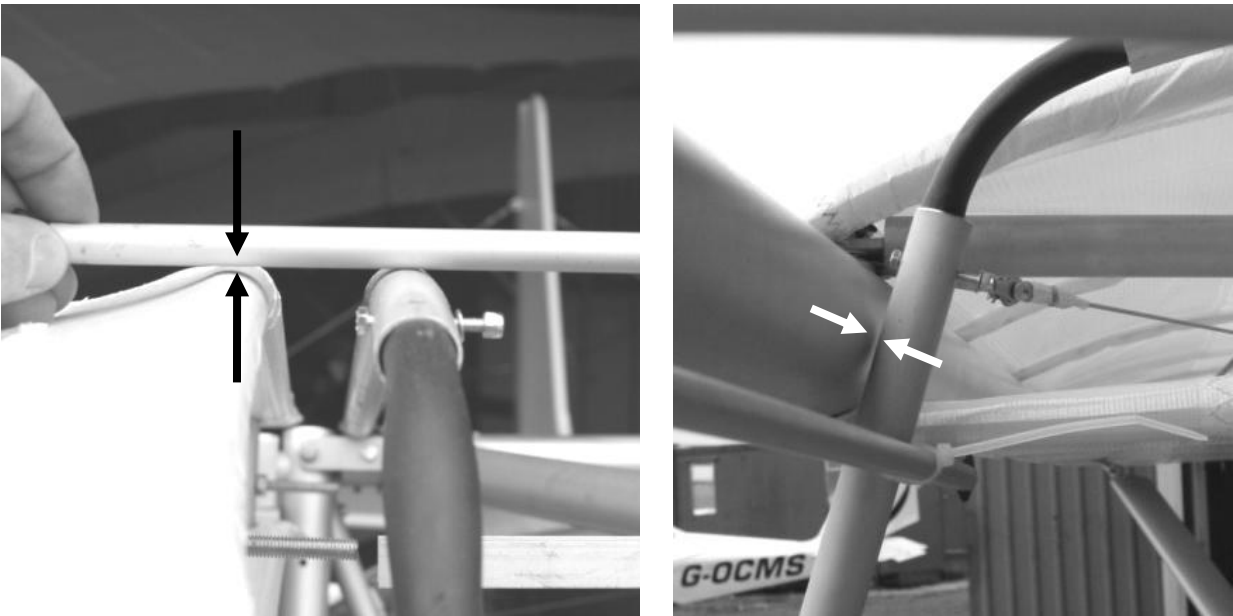
Figure 171 left – Check cabin roof tubes align with wing – level or slightly above. Right – check there is a gap of around 3-5mm here.
