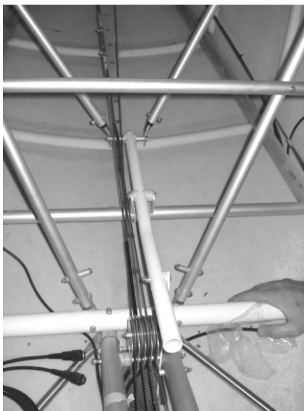
Figure 109 cable routing past flap handle.
