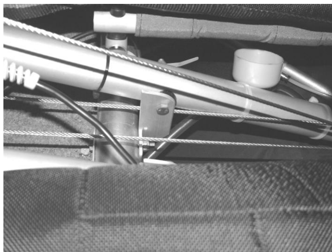
Figure 115 starboard rudder cable routing past central braces.
