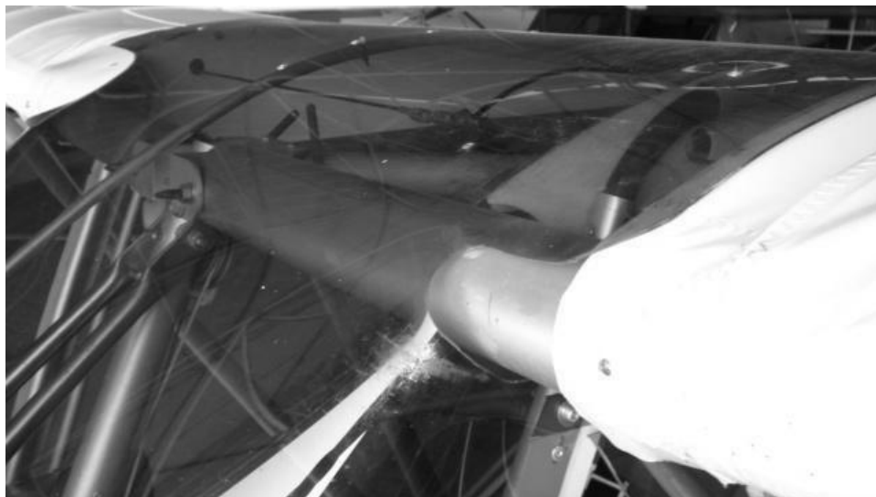
Figure 174 match up with wing so clear roof section will later fit flush like this
