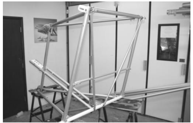
Twin TU19 tubes in position
