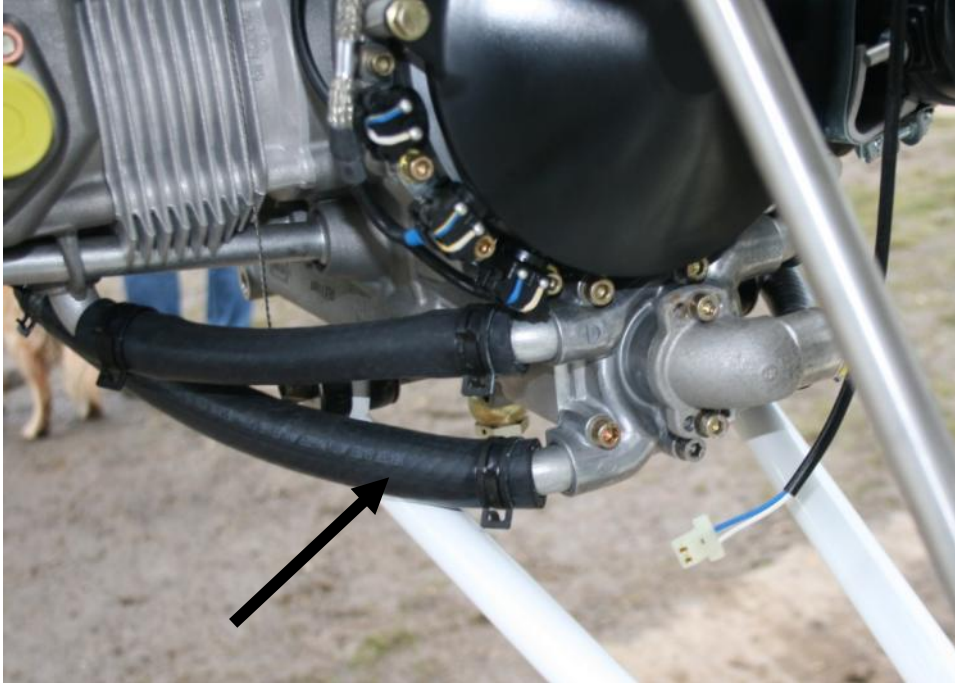
Fig 143 area of possible fouling between water pipe and lower engine mount
