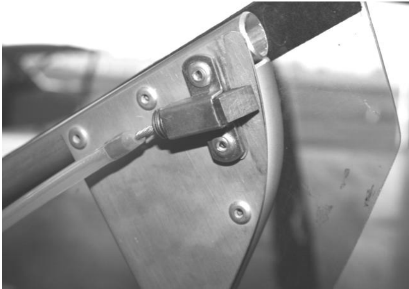
Figure 321 rear gusset plate and rear end of lower door.
