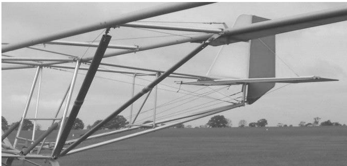
Figure 54 rear fuselage on uncovered frame.
